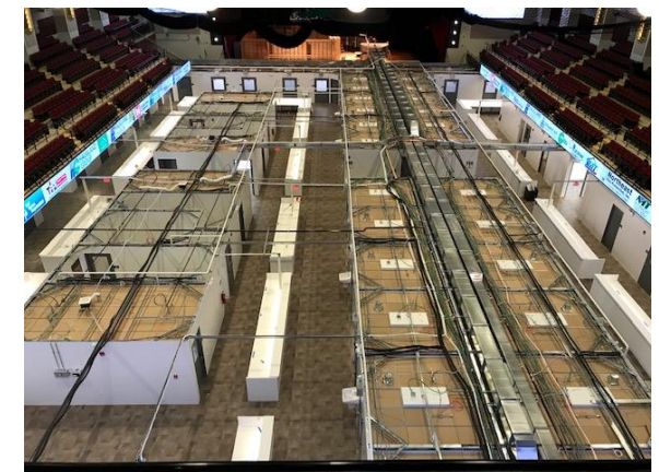
Interior Build Out
